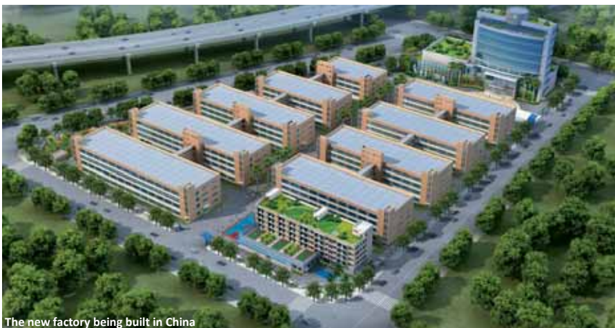
The new factory being built in China
